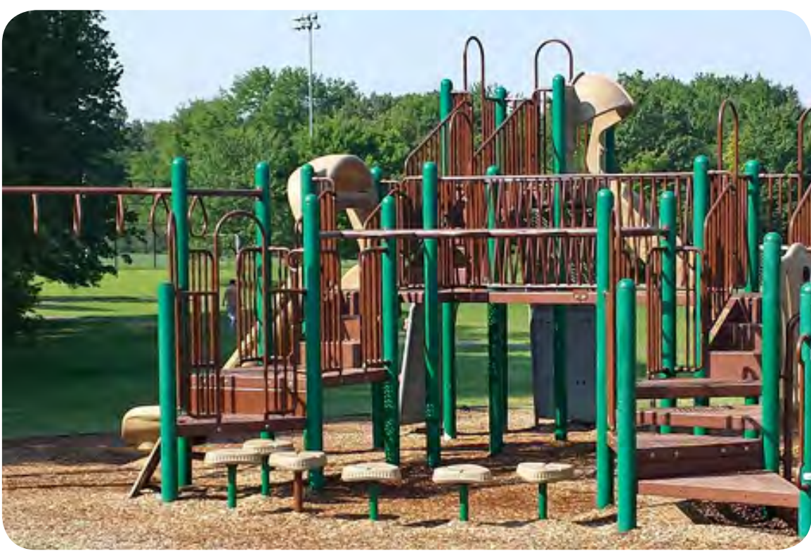
S-107 - Playground Structure
