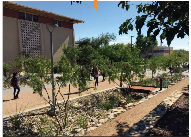
University of Arizona retrofitted their parking lot landscape buffer with a swale to capture runoff.
