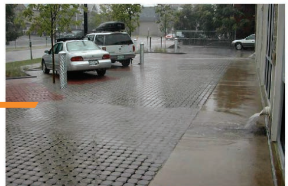
Permeable Pavement can capture most stormwater runoff.
