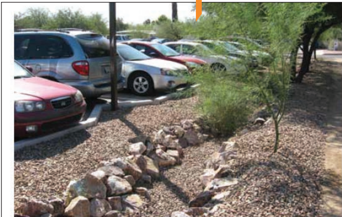
University of Arizona retrofitted their parking lot landscape buffer with a swale to capture runoff.
