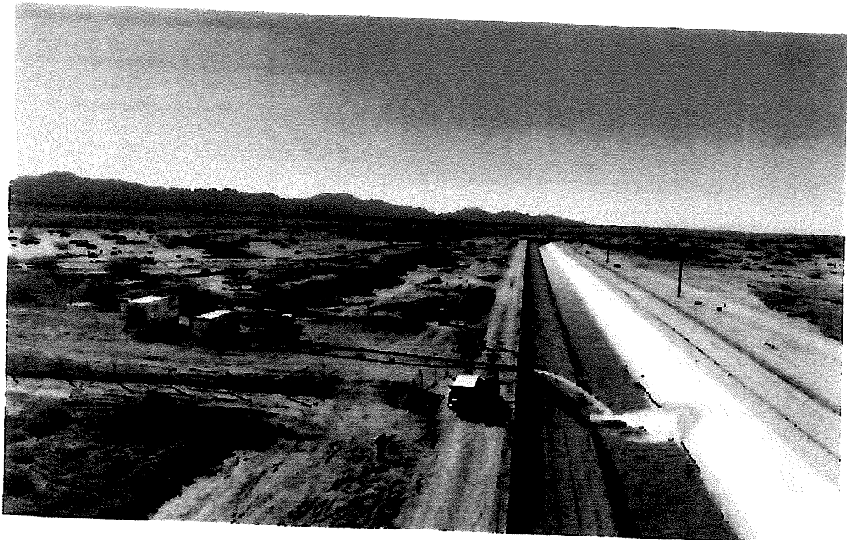
Test Pumping 4,900 GPM
