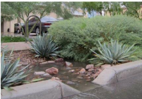
A Standard Curb Cut allows runoff to enter a lower landscaped area.
