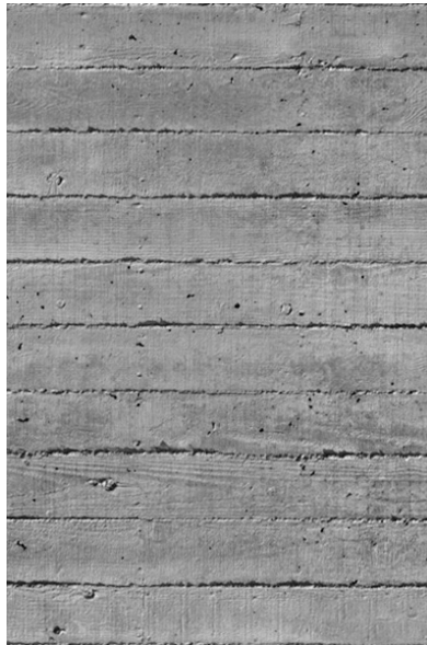
BOARD FORMED CONCRETE FEATURE WALL
