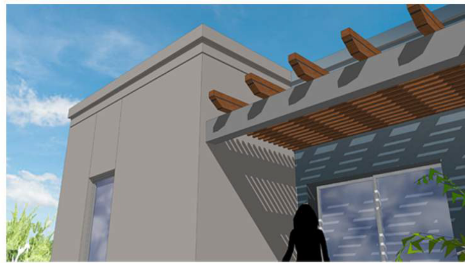
patio and window shade trellis
