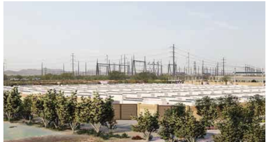
VIEW OF BATTERY ENERGY STORAGE LOOKING NORTHWEST
