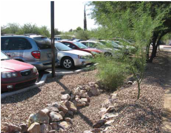
University of Arizona retrofitted their parking lot landscape buffer with a swale to capture runoff.
