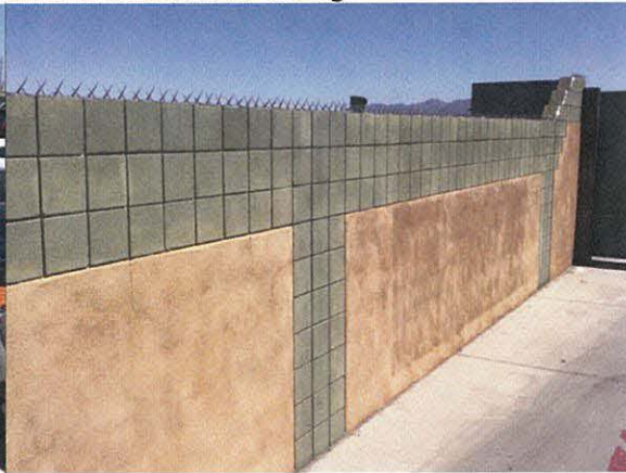
Structural Concrete Fencing
