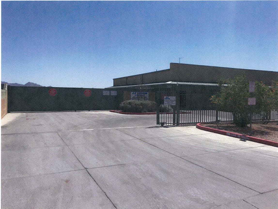
Main Entrance from Riley Drive
