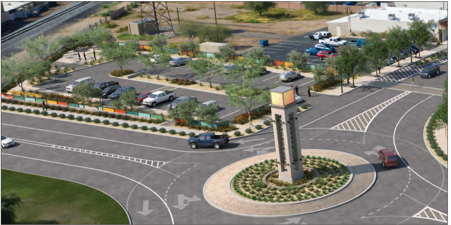
Figure 2-3 Southwest corner of Dysart Rd and Western Ave Parking Area
