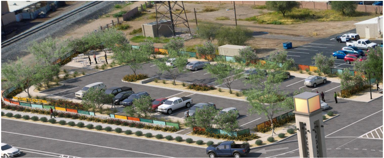
Figure 2-3 Southwest corner of Dysart Rd and Western Ave Parking Area
