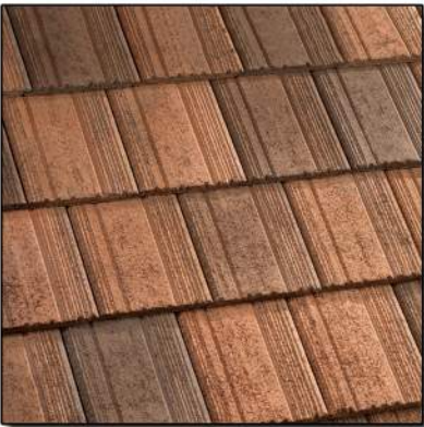
Roof Mfg: Eagle Roofing Golden Eagle 145 Sunrise Blend
