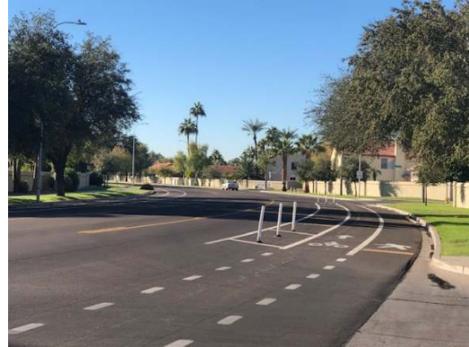
Figure 2b: Existing GPL near Emerald Lane
